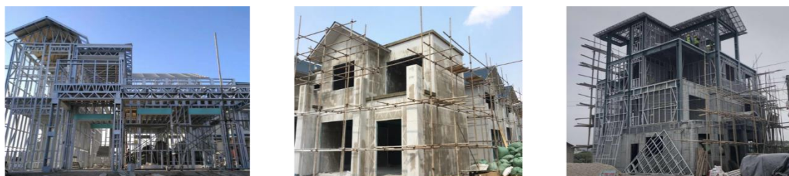
a) cold-formed thin-walled steel structure b) Light steel and lightweight concrete structure c) Light steel composite frame
